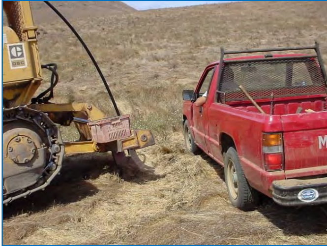
Figure 4. Rip shank and pipe feeder.
