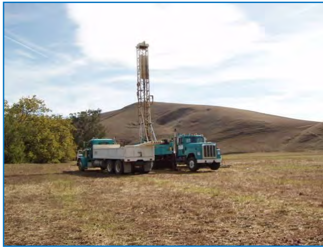
Figure 80. Site 1 well installation.
