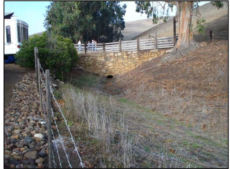
Figure 25b. Looking upstream at outlet and recontoured/revegetated banks.
