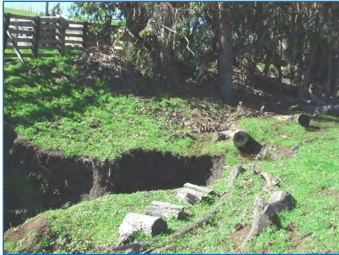
Figure 14. View of headcut, looking from left bank to right bank.
