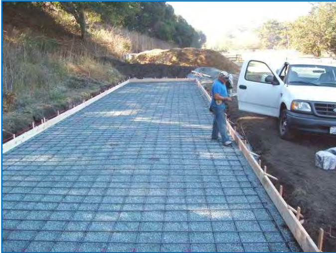
Figure 28. Contractor tying steel for pad.
