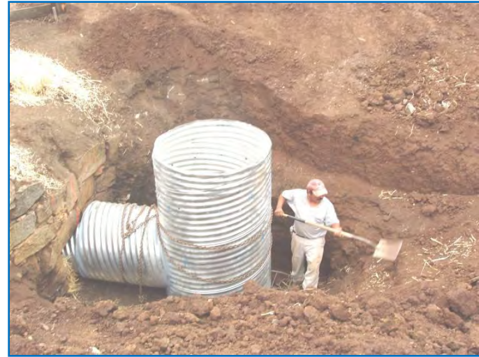
Figure 20. Placed drop structure.
