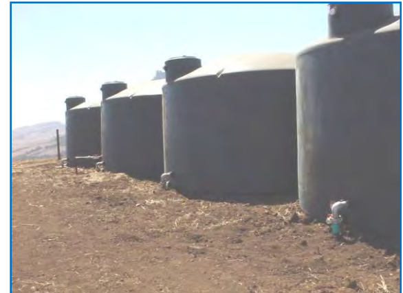
Figure 13. Four 5,000-gallon water tanks to supply troughs.
