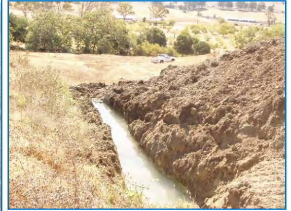
Figure 46. Development of lower spring in pasture 1.
