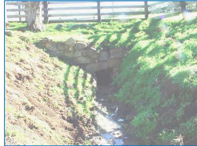
Figure 15. Looking downstream at entrance of existing rock culvert.
