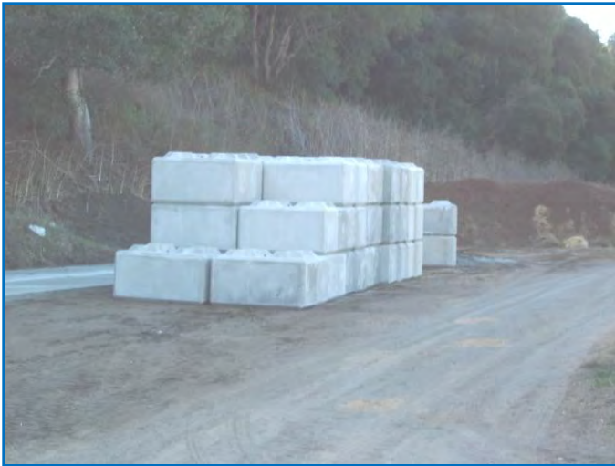
Figure 30. Inter-lock blocks off-loaded from truck, prior to placement on pad.
