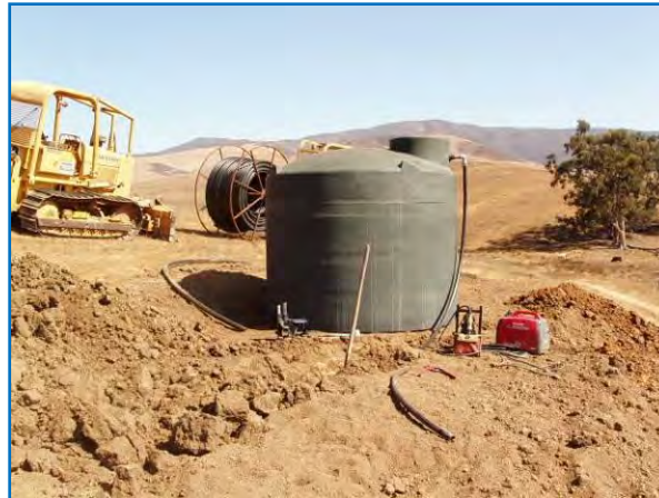
Figure 48. Installation of storage tank just below lower spring in pasture 1.
