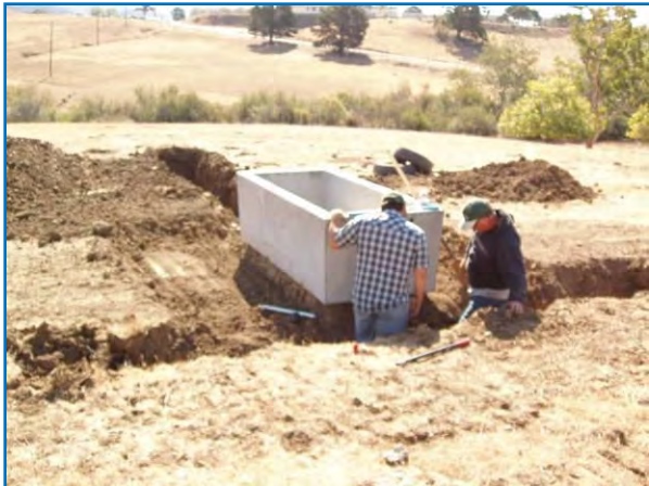
Figure 47. Installation of trough in pasture 5A.
