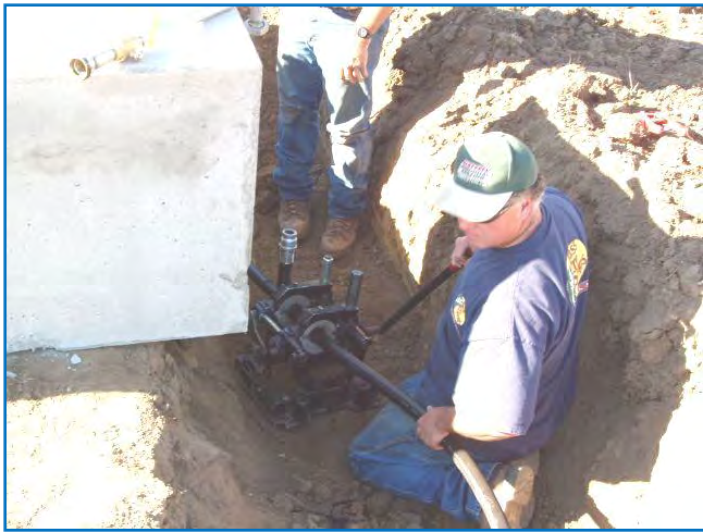
Figure 79. Installing tee to trough #30 with fusion welder.
