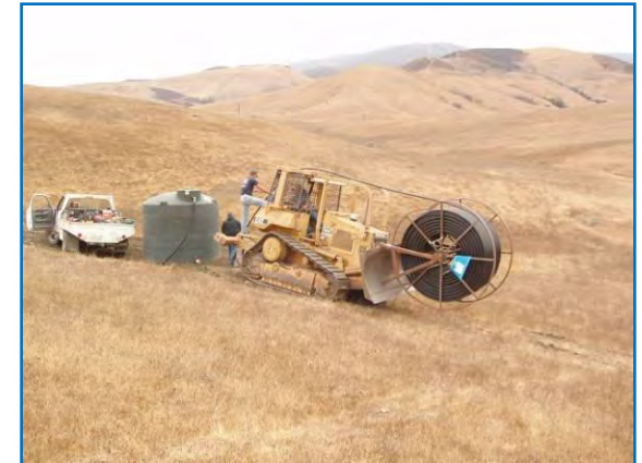
Figure 49. Installation of storage tank and pipeline to troughs in pasture 4.
