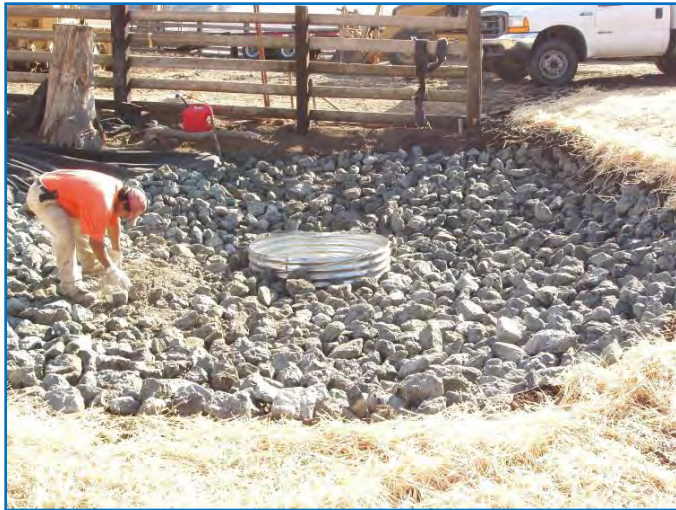
Figure 21. Looking downstream at riprap around drop.
