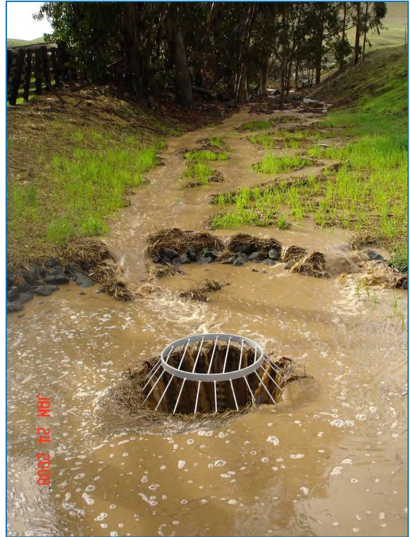
Figure 25. Looking upstream at drop structure and restored headcut during storm.
