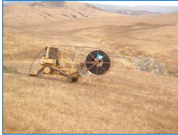
Figure 45. Ripping pipe in from upper spring in pasture 1 to trough.
