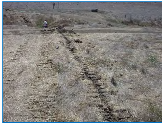
Figure 7. After pipe installation – minimal soil impact.
