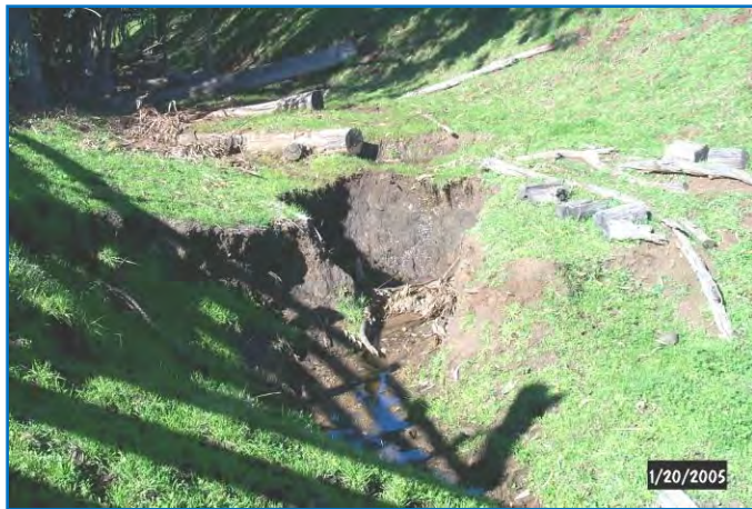
Figure 16. Another view of headcut.
