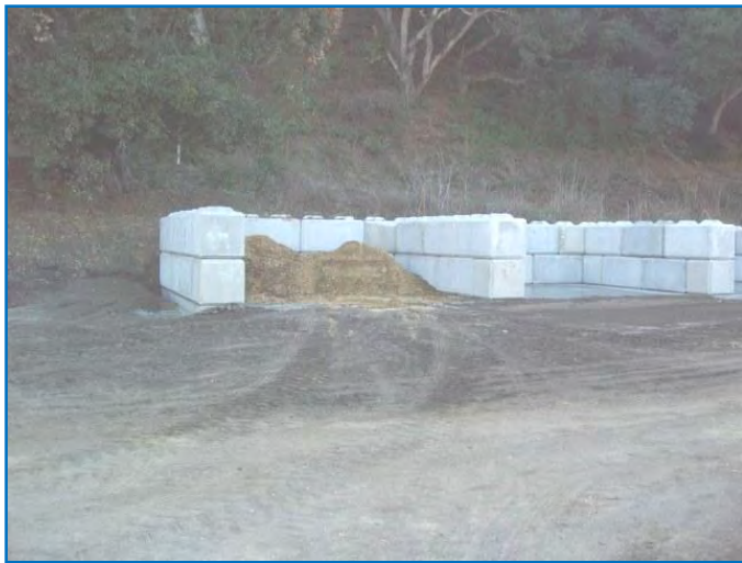
Figure 34. The first bin beginning to be filled with manure.
