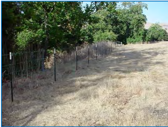
Figure 11. Installed fence along San Bernardo Creek.
