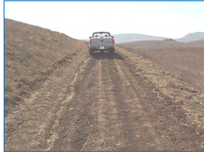
Figure 63. Developing gully in road.
