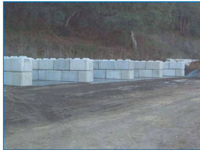
Figure 35. Closer view of 4 of 5 bins.
