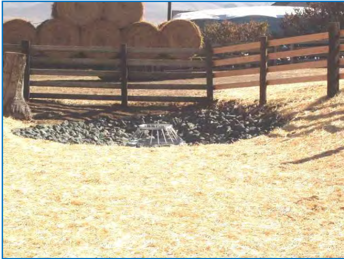
Figure 23. Installed drop structure and grate.
