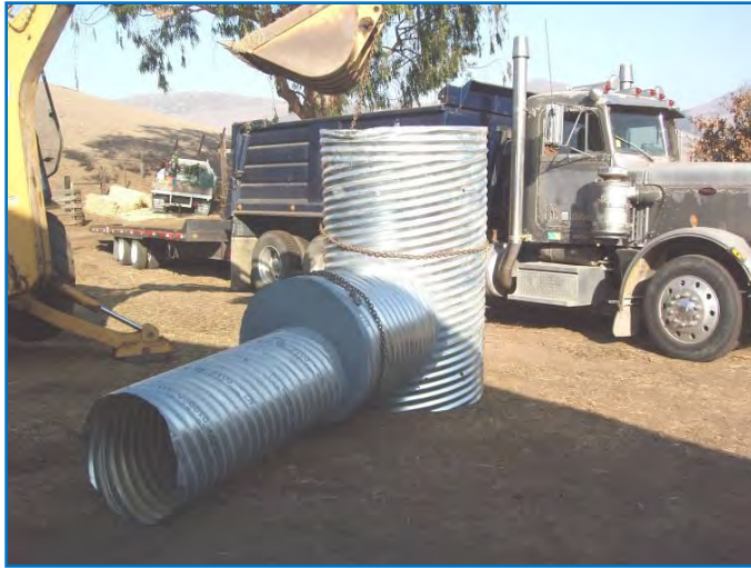
Figure 19. Drop structure prior to placement.
