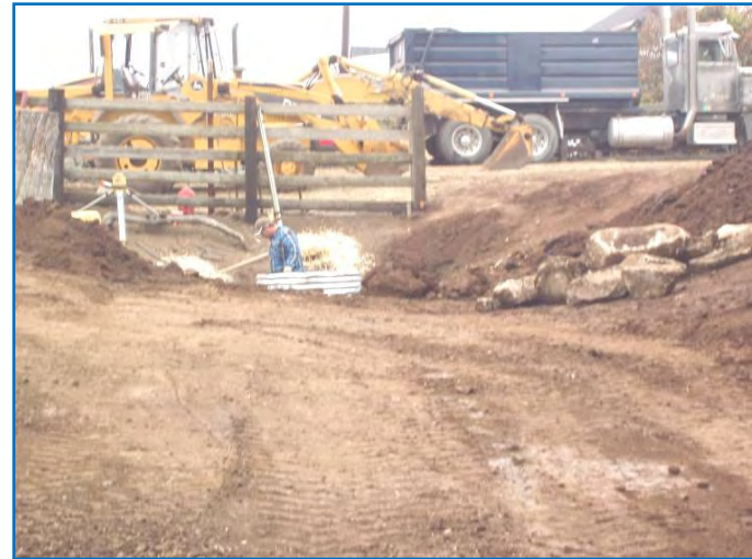
Figure 22. Headcut backfilled.
