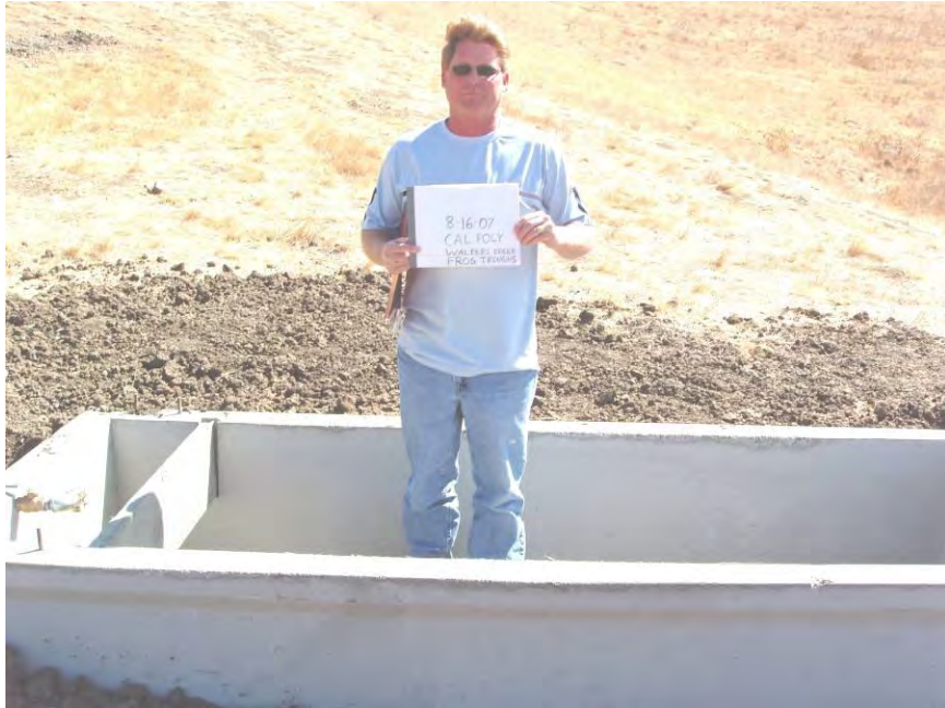
Figure 58. Trough in place in Walters Creek.
