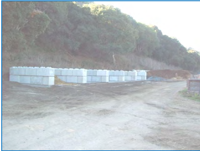
Figure 32. Blocks creating 5-bin compost facility.
