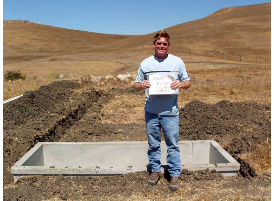
Figure 59. Trough set in place at Chumash Creek.
