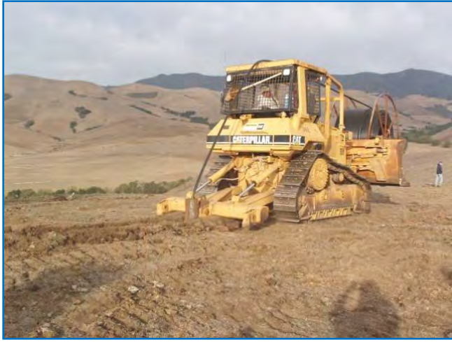
Figure 76. Cat and spool system used to rip in pipe.
