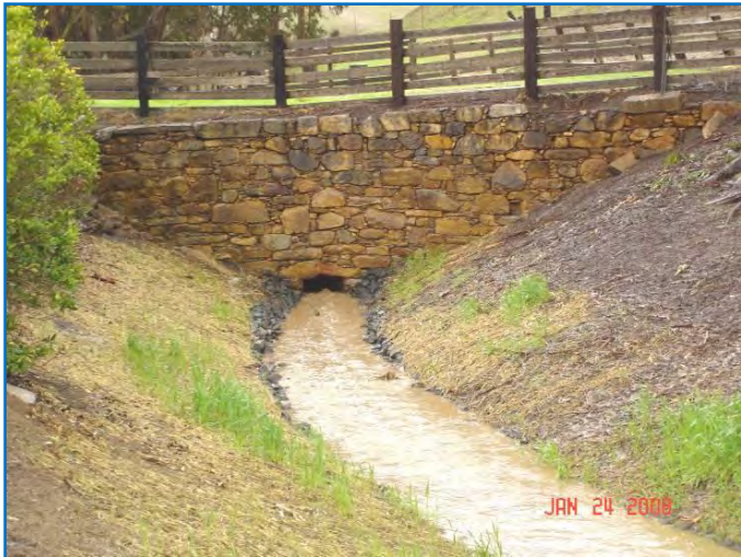
Figure 24. Looking upstream at outlet under stone bridge. Revegetated slopes are sprouting.
