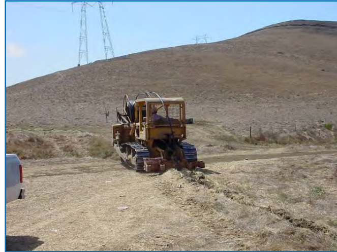
Figure 5. Close-up of cat ripping pipe into ground.
