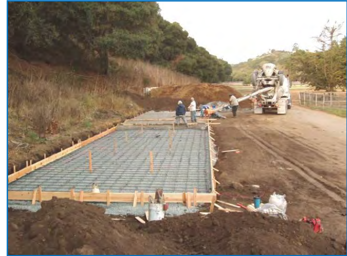
Figure 29. Pouring concrete.
