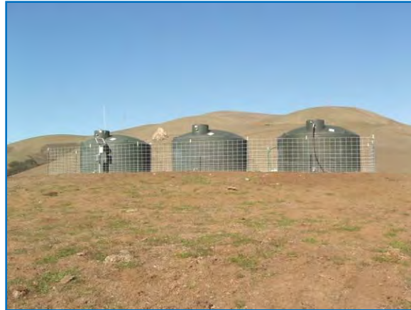
Figure 83. Three 4,500-gallon water tanks on north side of creek.
