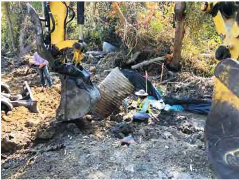
The existing culvert (left) was removed and a rocked ford was installed (below).
