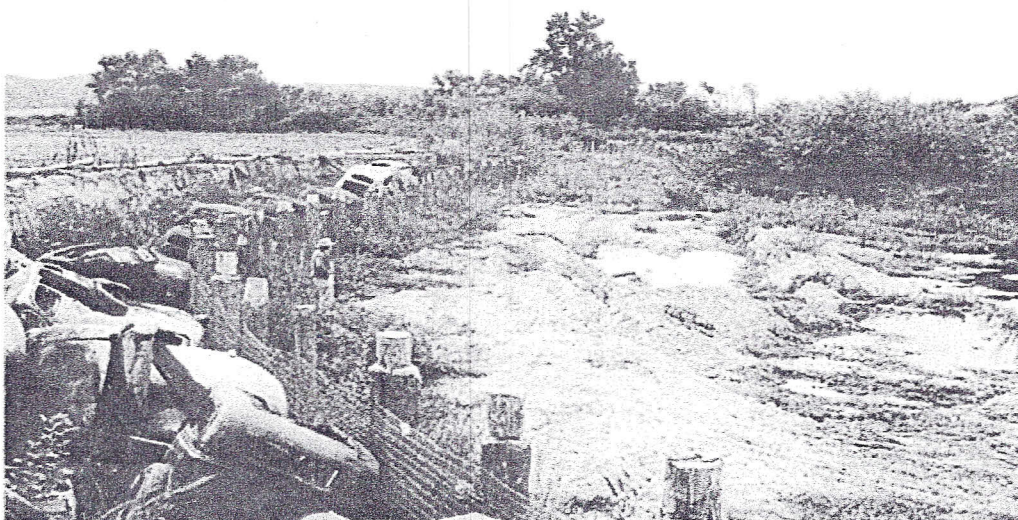
AG Creek after farmers made repairs-Clark Moore in picture on Vincent Antonio farm. 10/29/56
