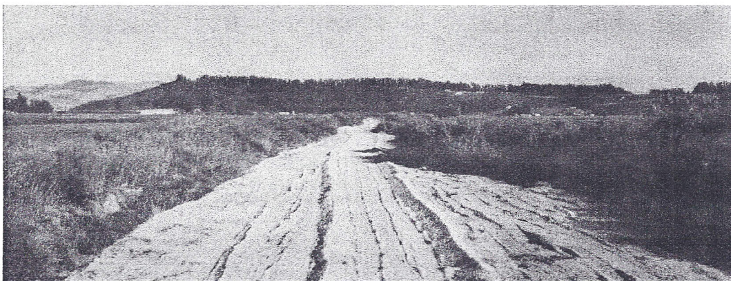
SLO County doing annual silt removal maintenance before 10/29/56.
