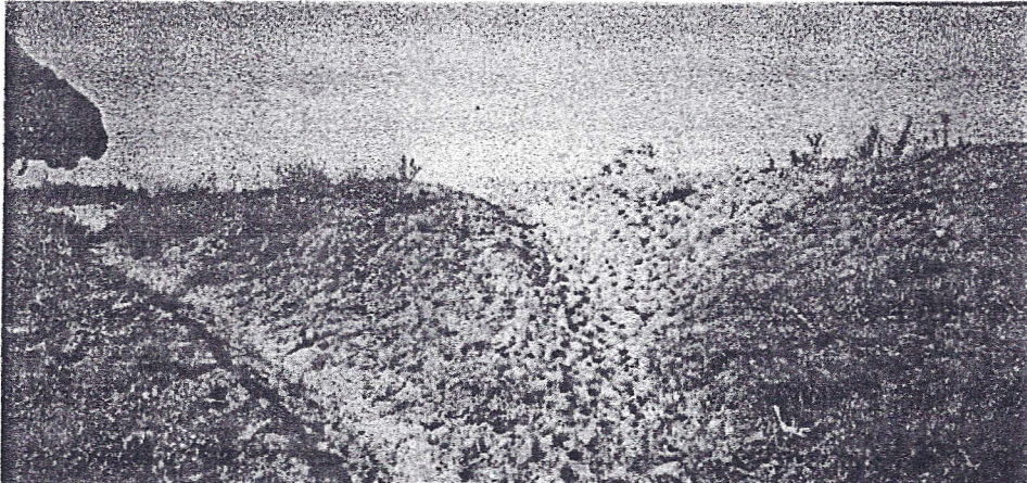
The Levees are used as riding trails and the picture documents the damage. Oct. 1999
