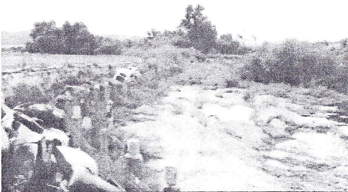
Inadequate Arroyo Grande Channel 1956
