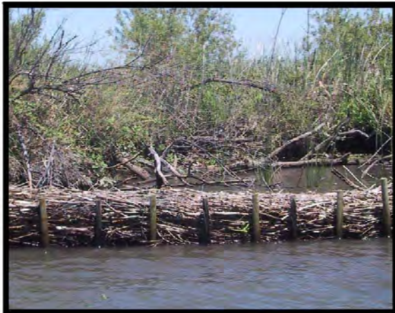
Branch box breakwaters, Option 2
