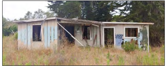
Photo 4: Primary elevation of the residence with the addition on the right, view facing west.
