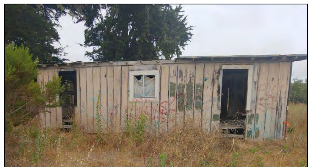
Photo 7: South elevation of the residence, view facing north.
