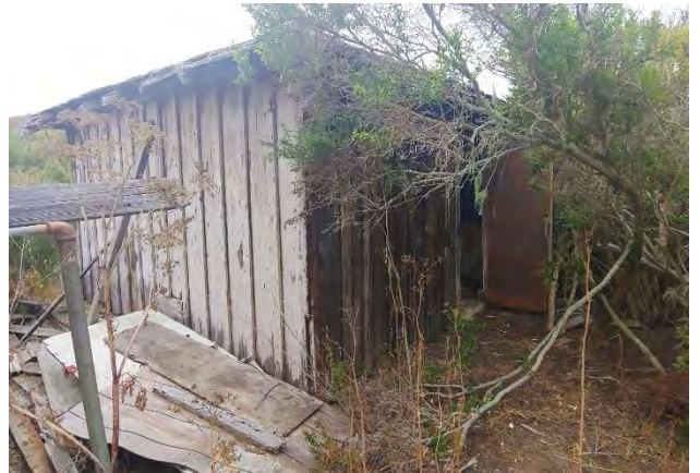
Photo 12: Shed exterior. View facing southeast.
