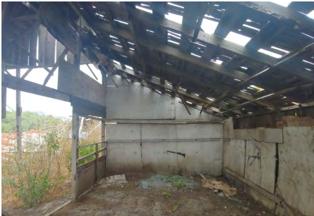
Photo 9: Crib on south side of barn interior, view facing east.
