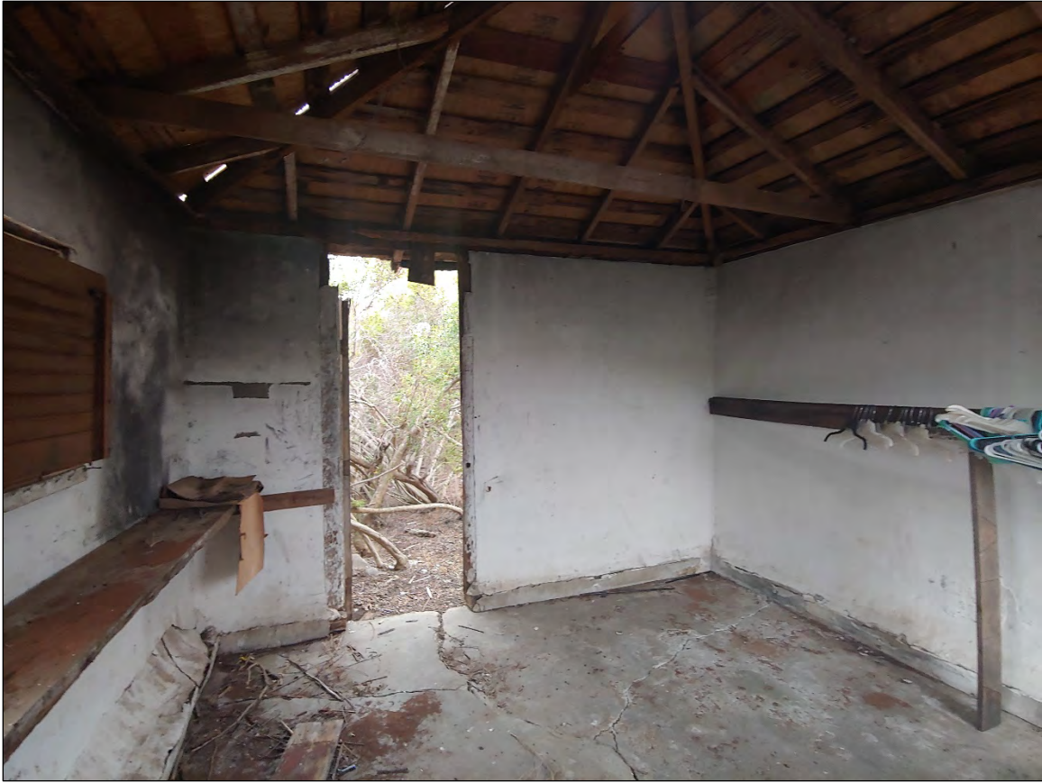
Figure 5-11 Shed interior. View facing west.
