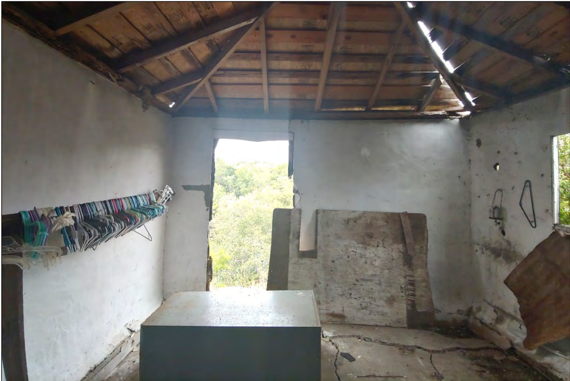
Figure 5-10 Shed interior. View facing east.
