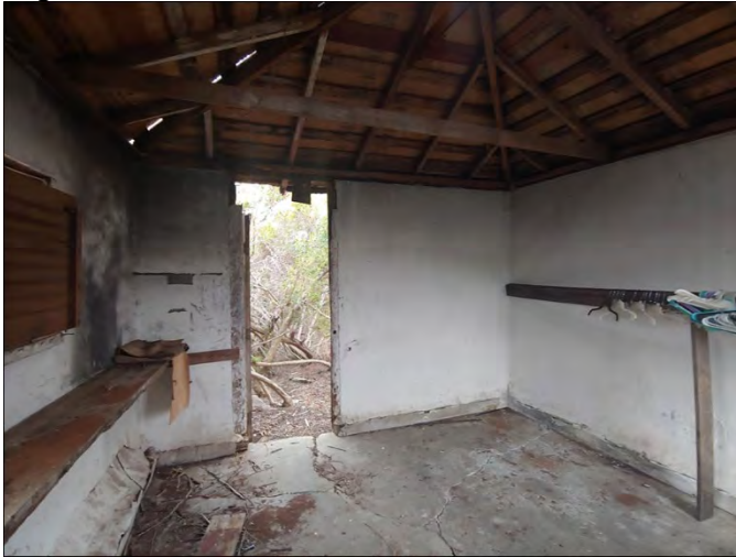
Photo 14: Shed interior. View facing west.
