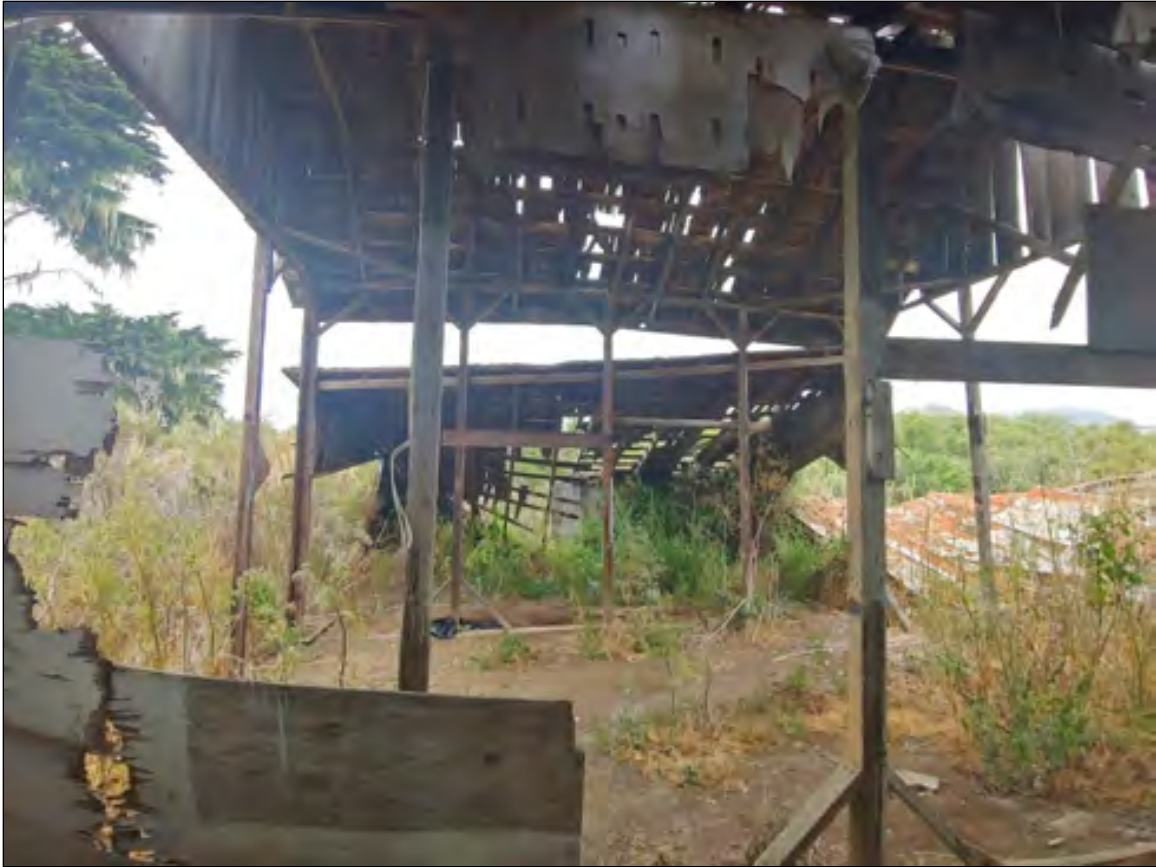
Figure 5-8 View from south crib barn interior, across barn, to north crib. View facing north.
