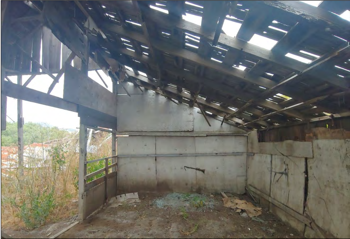
Figure 5-6 Crib on south side of barn interior, view facing east.
