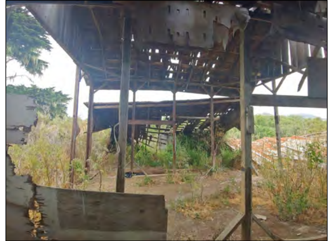
Photo 11: View from south crib barn interior, across barn, to north crib. View facing north.
