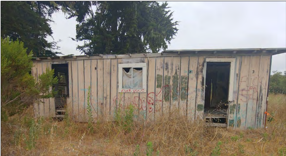
Figure 5-4 South elevation of the residence, view facing north.
