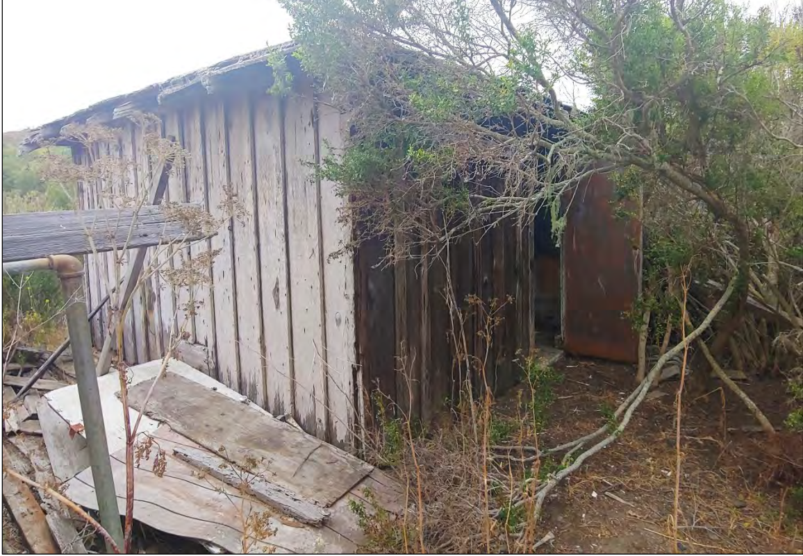
Figure 5-9 Shed exterior. View facing southeast.
