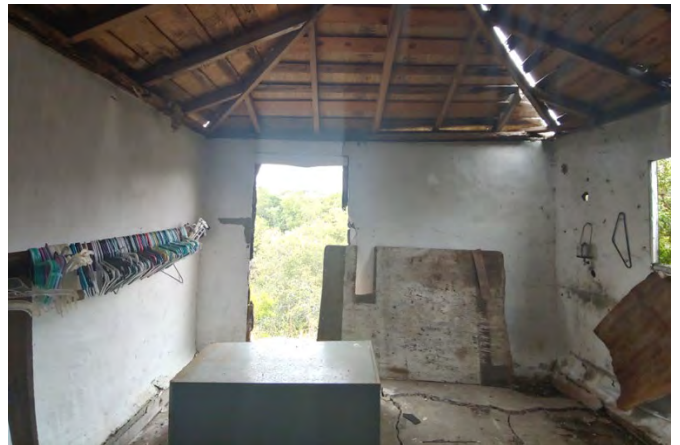
Photo 13: Shed interior. View facing east.
